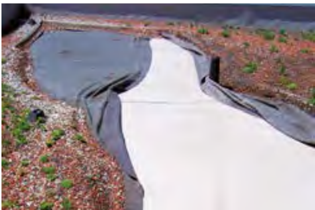
▲ Wind erosion, in this case all the way down to the roof waterproofing
